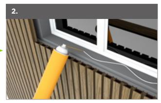
2. Secure the edge boards to vertical sides of window and also to underside (if sill not present or long enough) with both structural adhesive sealant and 35mm colour head screws.
