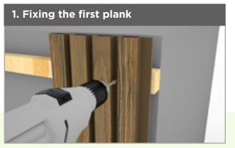
1. The first cladding plank will first need to be fixed with a 35mm colour head screw through the low 'valley' of the cladding profile.
