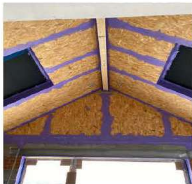
OSB board connections.
