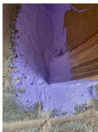
Joist connection on to masonry wall.
