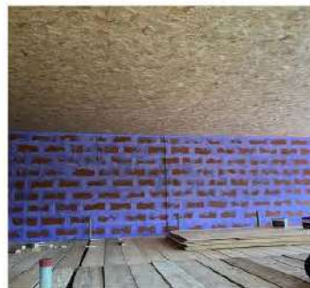
Passive Purple Brush applied to wood fibre.
