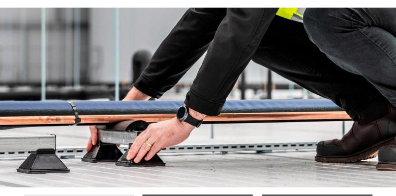
PVC Coated External Grade Insulation. External pipework needs to be insulated in a tough PVC coated weather protected covering to avoid UV degradation and animal damage.
