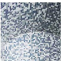
This board has grooves cut into one surface that make it flexible allowing it to be flexed into curves and even circles. Once fixed to a wall or a frame the board provides a strong solid substrate for tiling or plastering. The board can be fixed
